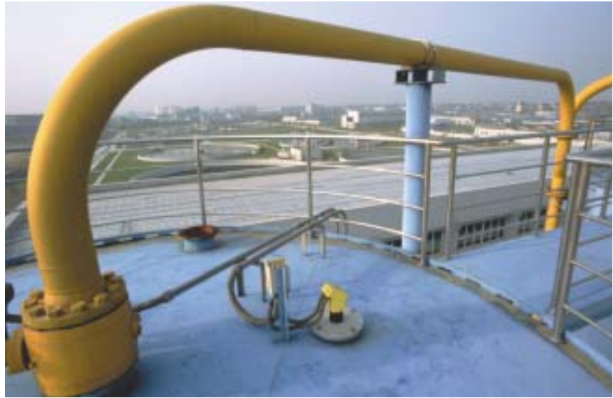
Silo roof with filler line, ventilation connector and ultrasonic sensor for measuring the filling level
