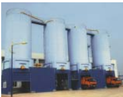
4 Silos each with a volume of 250 m 3 and 5.5 m diameter for loading onto heavy goods vehicle
