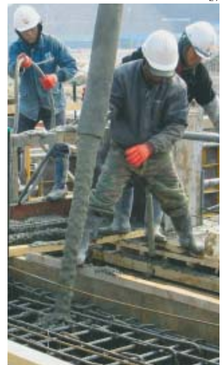
A saturated jet of concrete with a slump dimension of 12 cm
